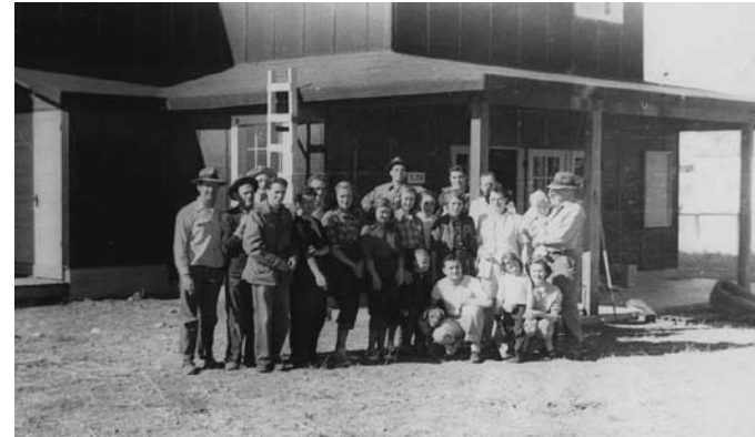
Gowen Field Theater with work crew
